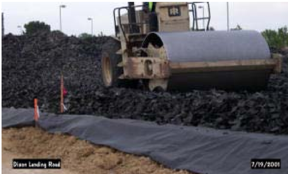
FIGURE 4. Dixon Landing Interchange Embankment Fill, Compacting TDA (12)
