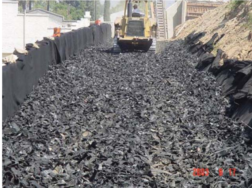
FIGURE 7. TDA as Backfill for Retaining Wall 119 in Riverside, CA (22)
