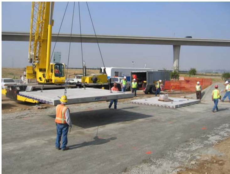
Figure 3. The construction the HVS testing-site for the precast pavement rehabilitation for the I-15 Ontario project.
