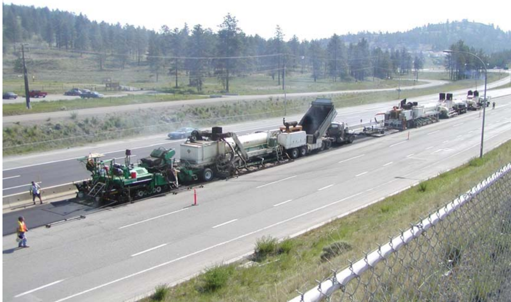
Figure 4 Multi-stage HIR train developed and manufactured by Artec and Pyrotech, but currently operated as the ARC Supertrain in British Columbia
