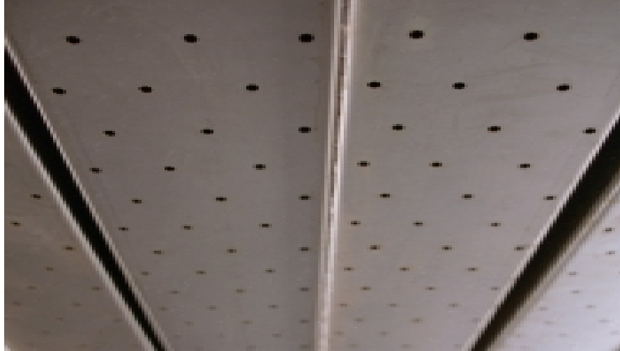
Figure 8 Close-up of the underside of the AR 2000 hot air heating system.
