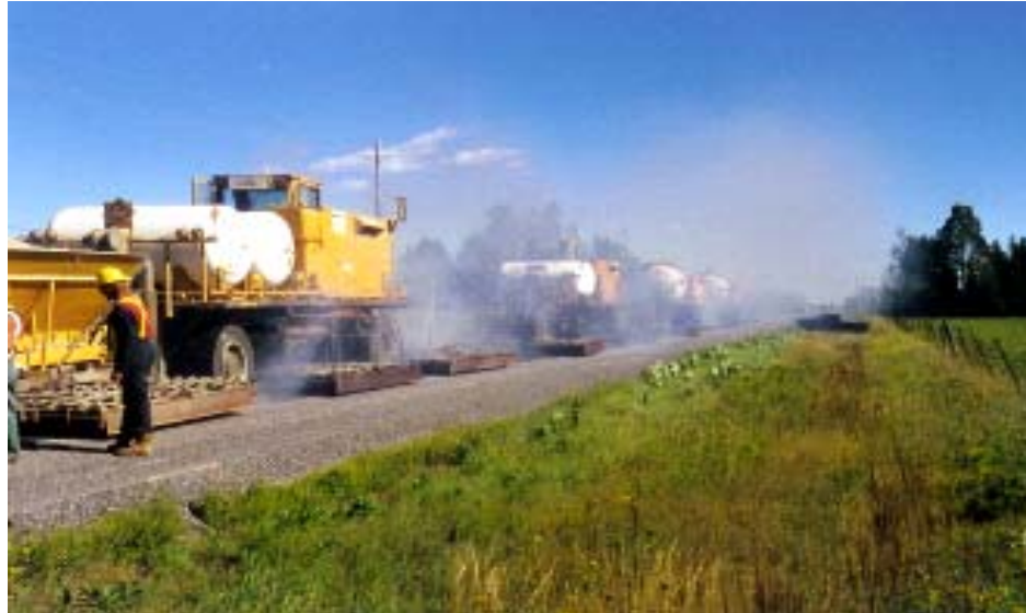
Figure 9 Example of HIR project with smoke being produced at an unacceptable level, indicating some overheating of the asphalt binder.
