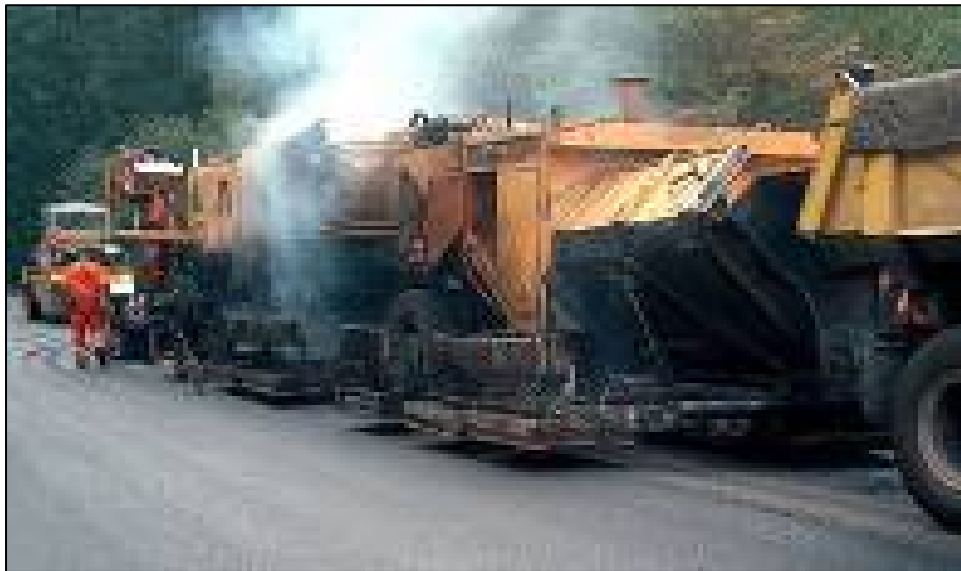
Figure 9 Example of HIR project with smoke being produced at an unacceptable level, indicating some overheating of the asphalt binder.
