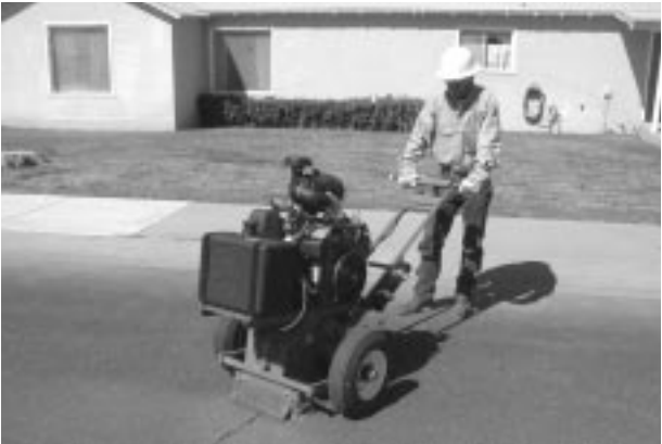
Figure 6.2. Router used to shape sealant reservoir for cracks.
