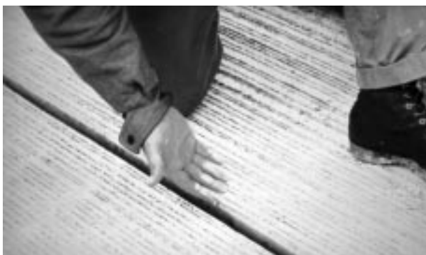
Figure 7.3. Dust and debris in a joint (or crack) will prevent proper adhesion.
