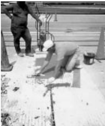
Figure 13.3. Finishing the patch surface.
