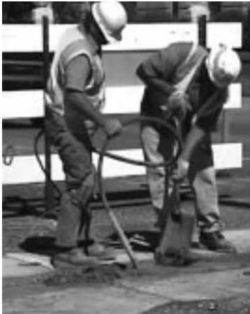
Figure 13.2. Consolidation of the repair material by vibration.
