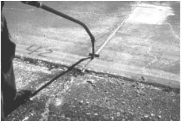
Figure 13.5. Resealing joints after partial-depth repairs complete.
