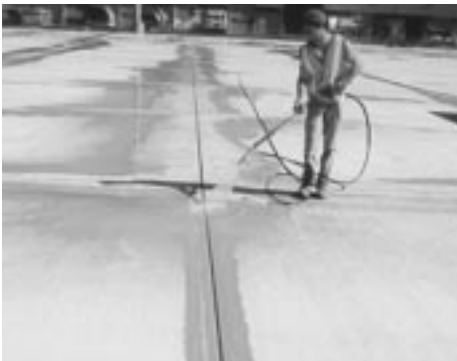
Figure 6.4. High-pressure water cleaning.
