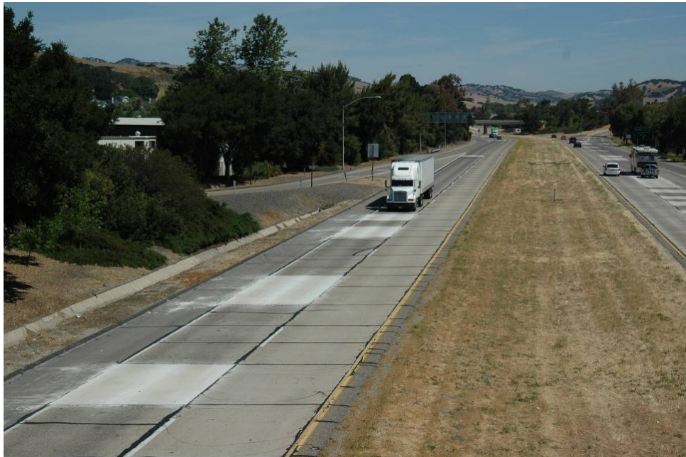
Figure 5. Panels open to traffic.
