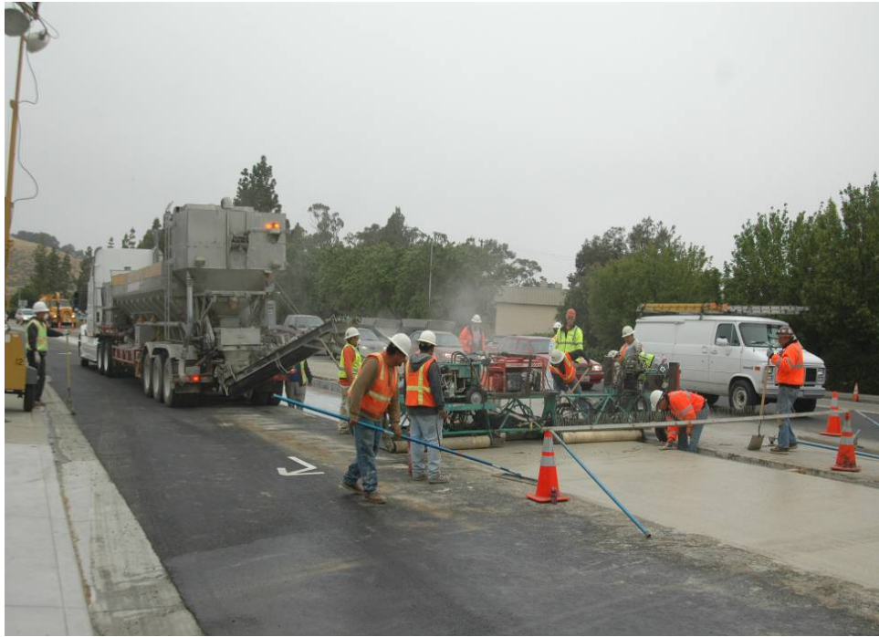
Figure 4. Finishing the panel.
