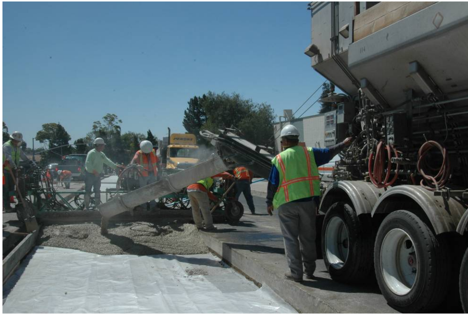
Figure 3. Mobile Mixer placing very early strength (VES) concrete.
