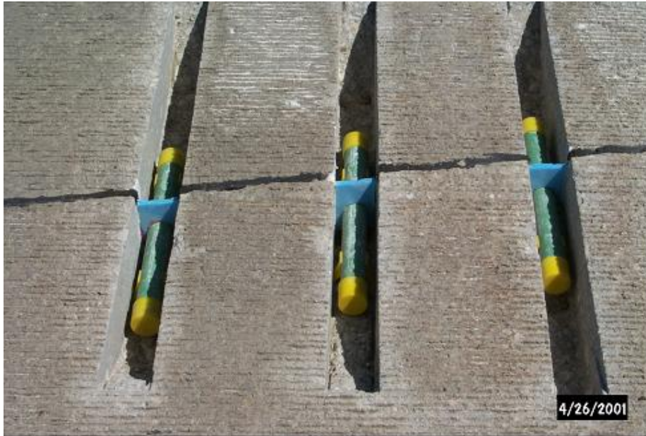
Photo 10. Retrofit dowel assemblies placed in the slots prior to backfilling.
