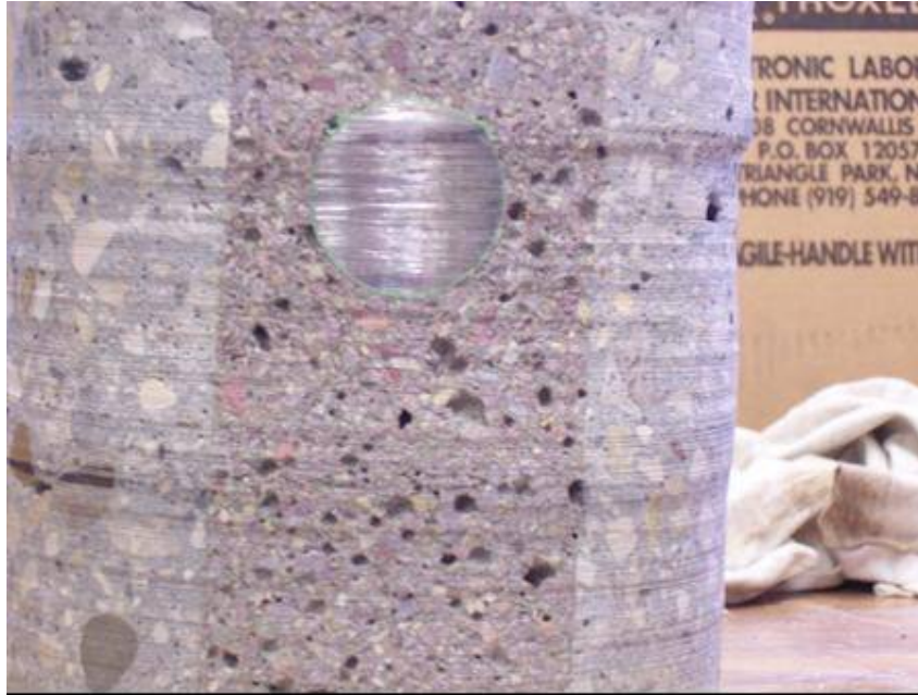
Photo 9. Core from TH 59 test site showing honeycombed retrofit mortar.
