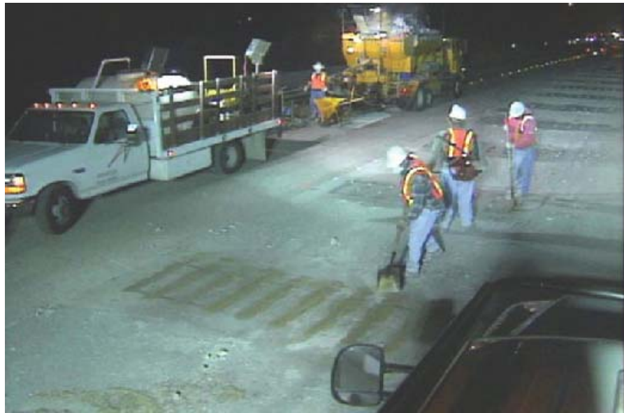
Figure 6. Successful dowel bar retrofit project on I-10 in Pomona, CA (9).
