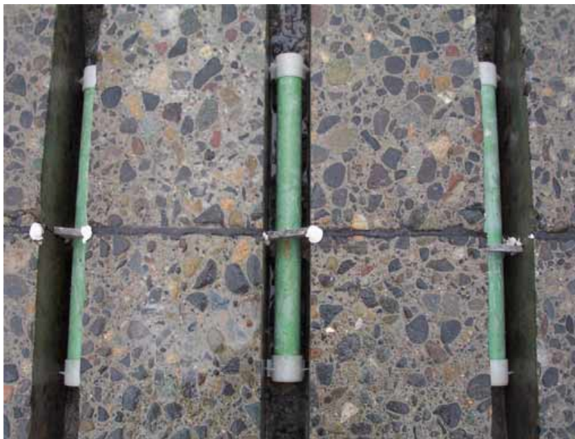
Figure 5. Dowel bar retrofits at a transverse joint (8).
