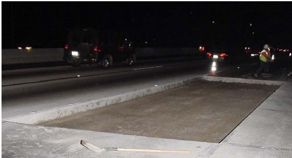
Figure 8. A full-depth concrete slab replacement project (11).
