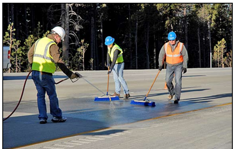
Sweeping in the Sealant on I-80
