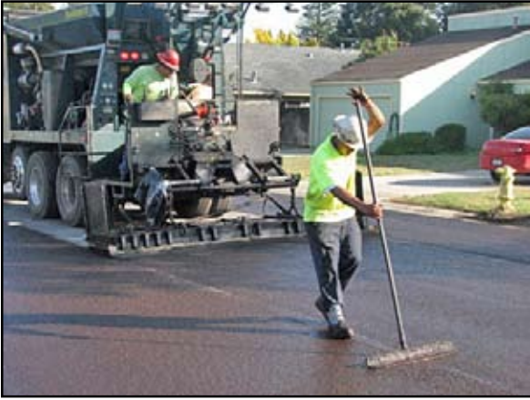
Workers place micro-surfacing over scrub seal on a residential subdivision street
