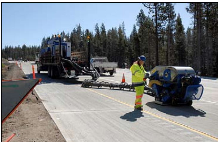
Test section on I-80
