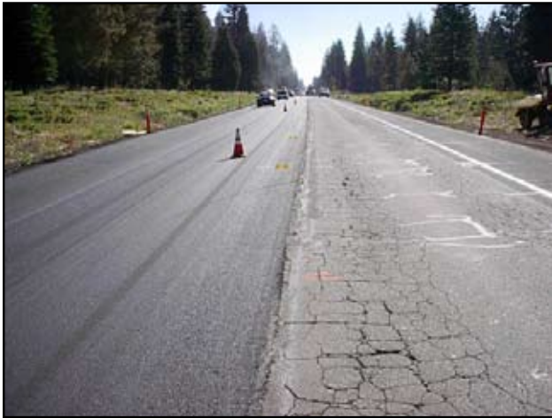
Before and after construction on SR 36
