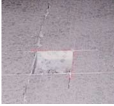
The prepared area, clean and ready for the patch material.
