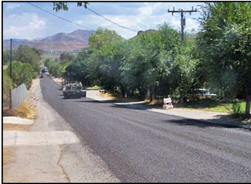
Finished chip seal surface.
