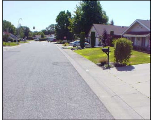
Hidden Hills Rd before rubber cape seal
