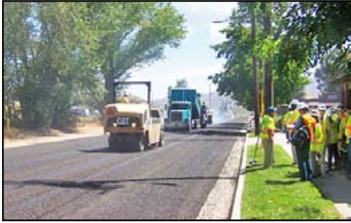
Spray application, rock spreader and compaction.
