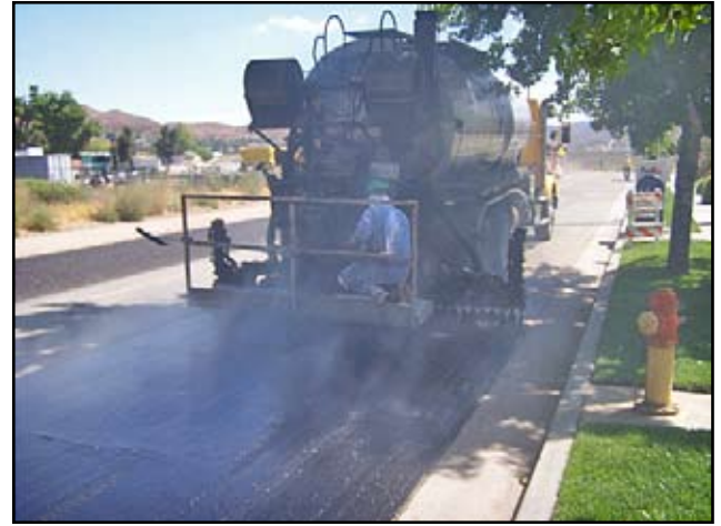
Warm mix asphalt rubber spray application. Notice the lack of smoke.
