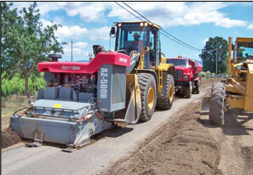
FDR with Lake County's Asphalt Zipper
