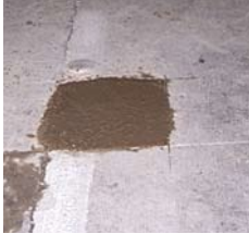
Patch material in place, I-10 east-bound lanes.
