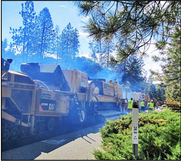
Field testing of recycling train
