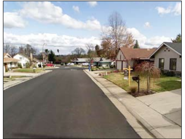
Hidden Hills Rd completed rubber cape seal
