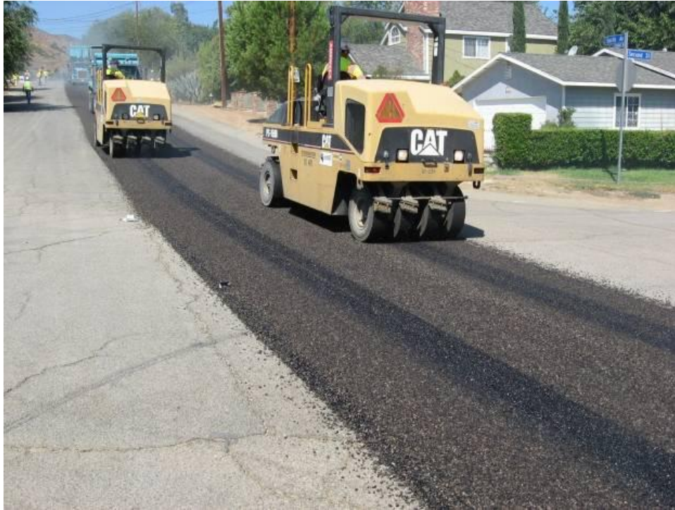
Figure 7 Compaction
