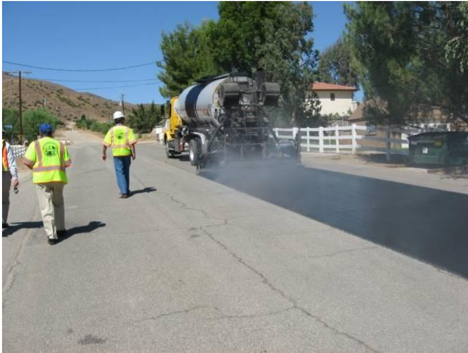
Figure 8 Visible emissions during binder application
