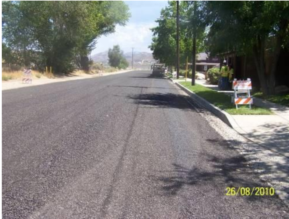
Figure 50 Finished chip seal
