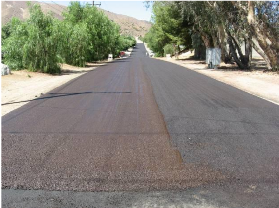
Figure 7 Finished cape seal on Smith Avenue
