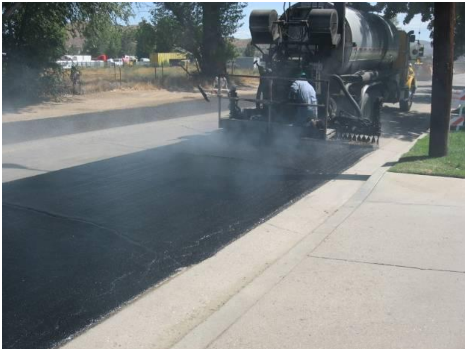
Figure 4 Emissions during binder application
