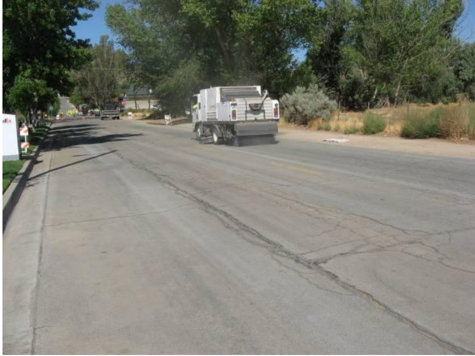
Figure 4 Sweeping the existing surface before laydown of AR chip seal
