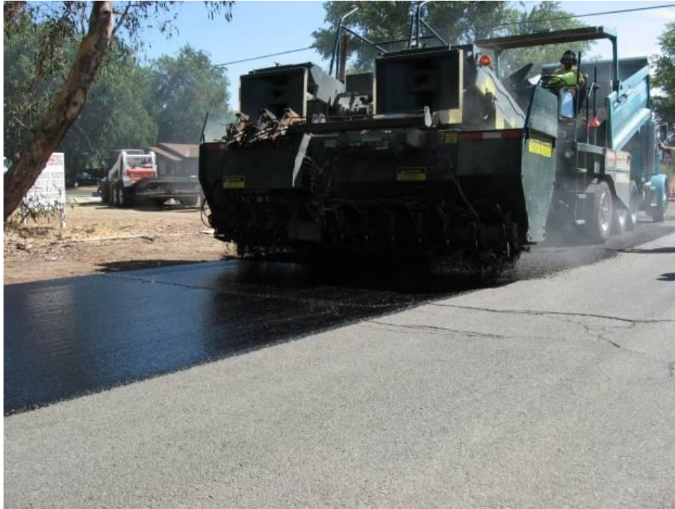
Figure 6 Chips placed on the asphalt rubber binder with warm mix additive
