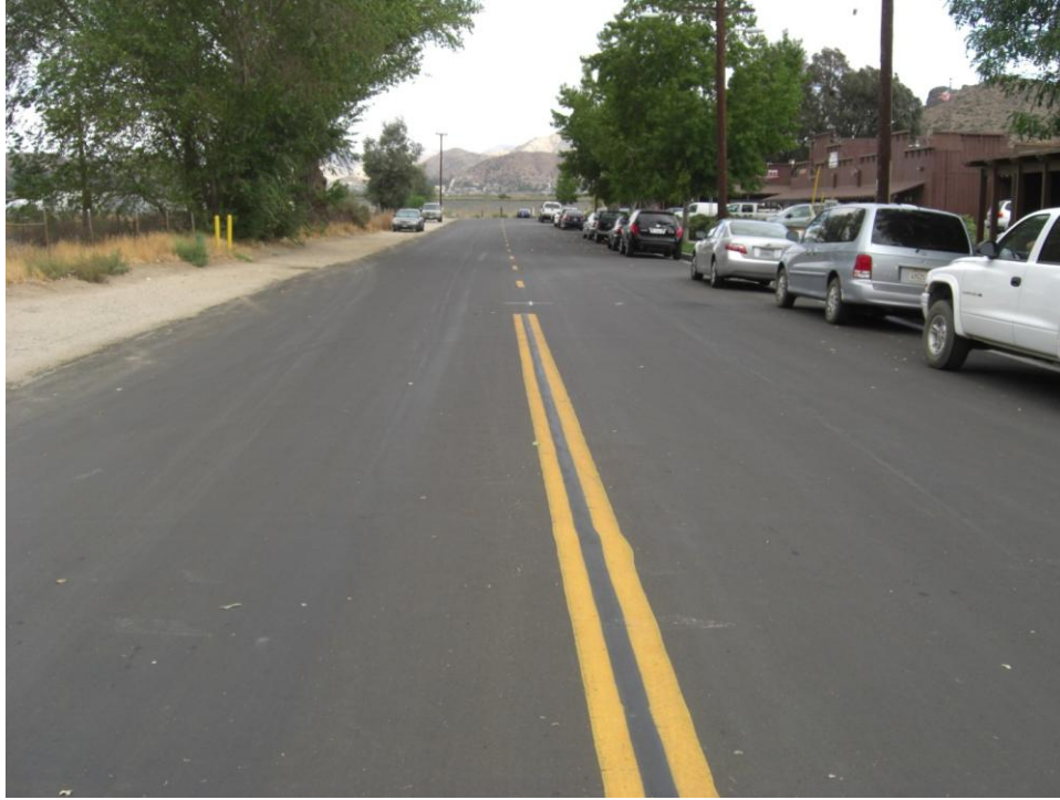
Figure 13 Smith Avenue after striping
