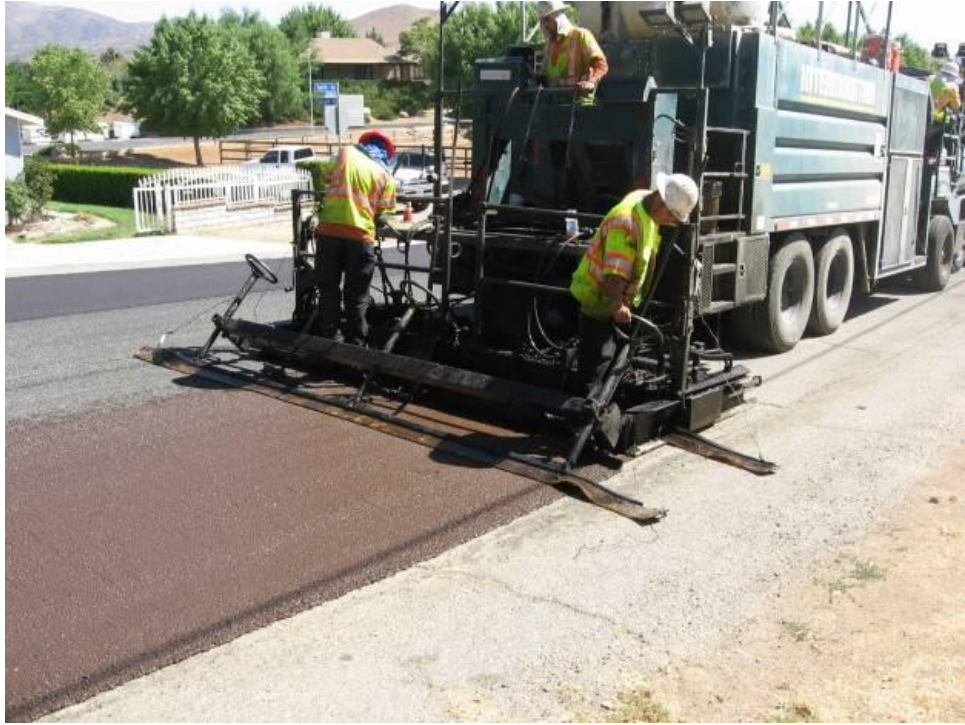
Figure 6 Microsurfacing applied over chip seal
