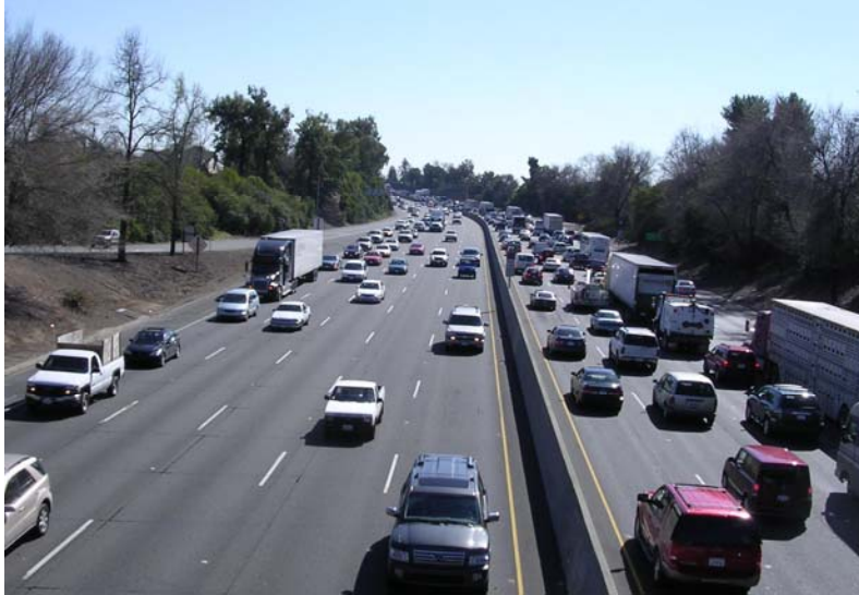
Sutterville Overpass Looking South
