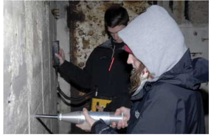
Fig. 4: Inside the observation post, Courtney Sheehan tests relative concrete strength with a Schmidt (rebound) hammer while Chad Golden uses a cover meter to determine location, size, and cover of embedded reinforcing
