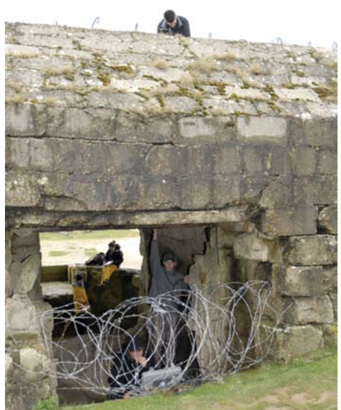
Fig. 7: Chad Golden (on top of the casemate) holds a transmitter that is sending ultrasonic pulses through the approximately 2 m (80 in.) of concrete to where Robert Hostettler (inside) is holding the receiver. Andrew Billingsley (seen through the barbed wire) is running the test data via a field-ruggedized computer on the velocity of the sound waves to determine soundness of the concrete
