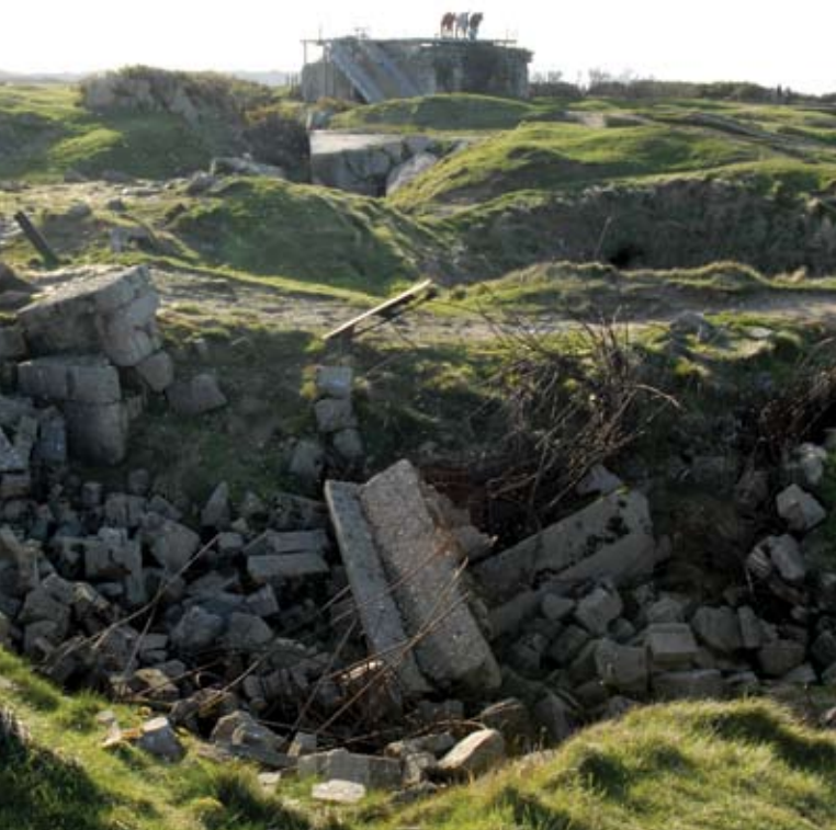
Fig. 6: Casemate that appears to have been under construction at the time of the D-Day invasion and was destroyed by a bomb prior to completion. The sack of hardened cement in Fig. 5 sits nearby
